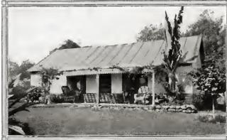
Six Rooms and Bath Comprise This Tent-House Which Cost \$630. The Walls are Constructed of Clapboards and Duck
